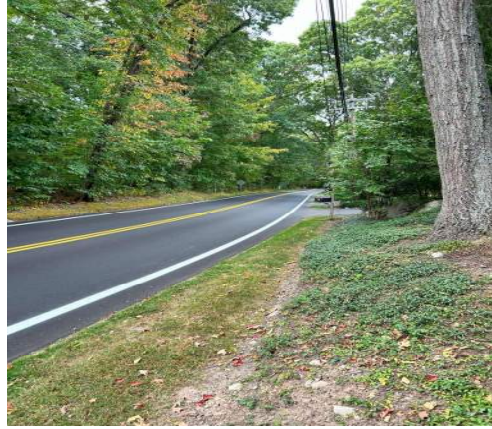
Northbound School Zone
