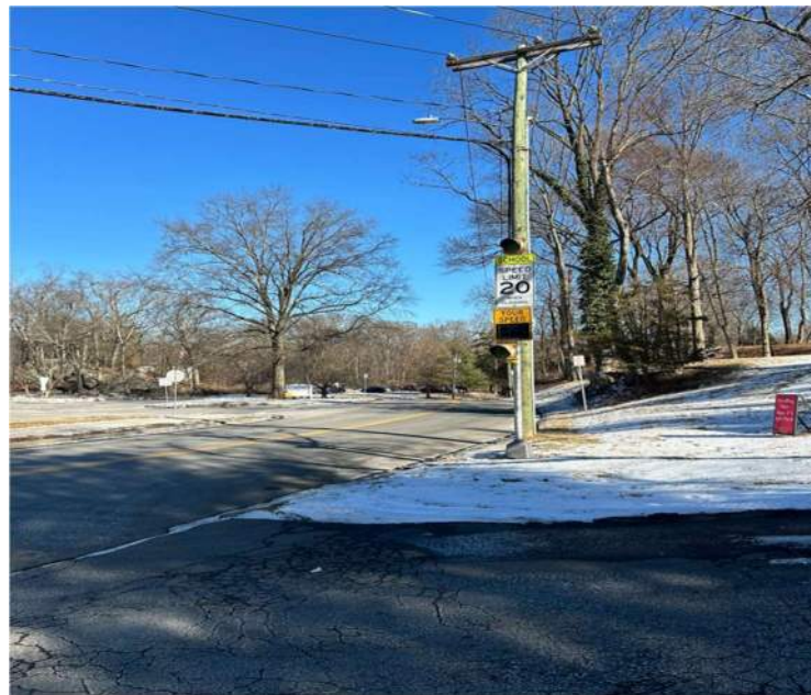
Eastbound School Zone Flasher
