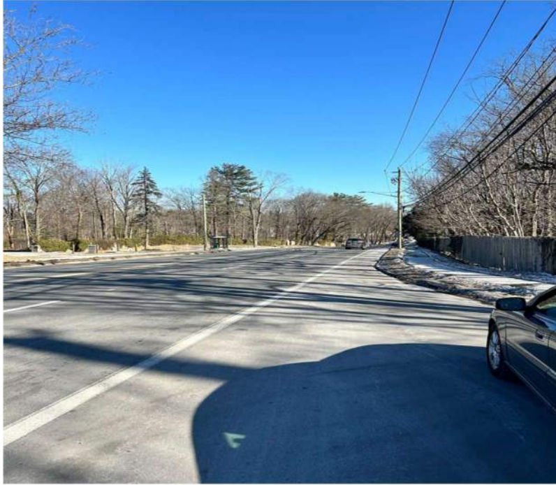
School Zone Eastbound
