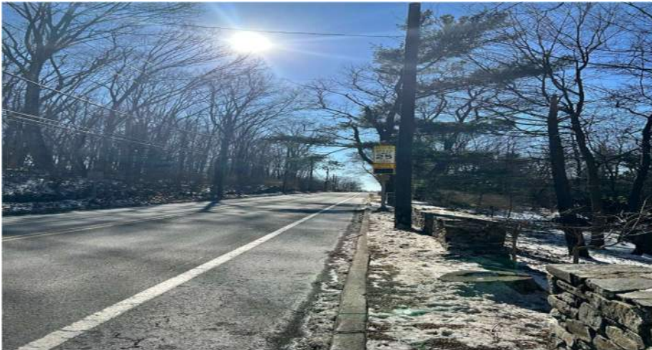
Southbound School Zone Flasher
